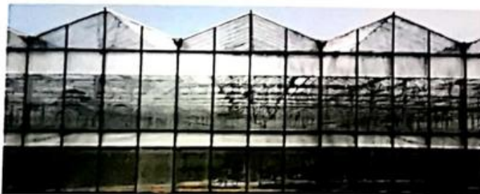
Figure 3.11 A modern greenhouse. Built on an aluminium frame, the sides are constructed of glass and the roof of double-walled polycarbonate (which is stronger and a better insulator than glass). The mixture of glass and polycarbonate mean this cannot be described as a 'glasshouse'.
