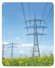
▲ Electricity cables: aluminium (light) with a steel core (strong).
