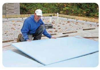
▲ Polystyrene is an insulator: it helps to prevent heat loss. So it is used under floors, and in fast-food cartons.
