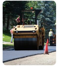
▲ The new road surface is bitumen mixed with fine gravel.
