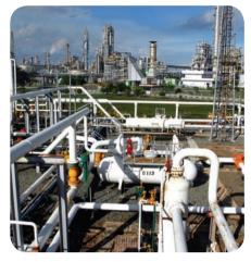
▲ Ammonia plants are often built close to oil refineries, to make use of the hydrogen from cracking
